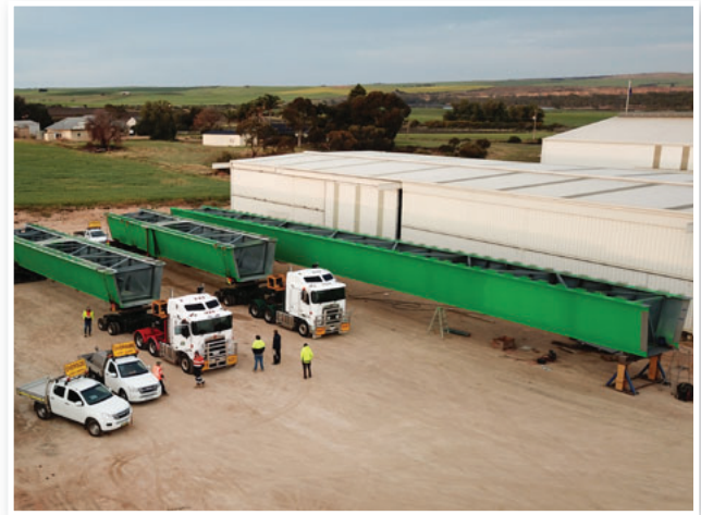
R2P Road Project - Bridge Girders “The first girder segments ready to leave the manufacturing site”
