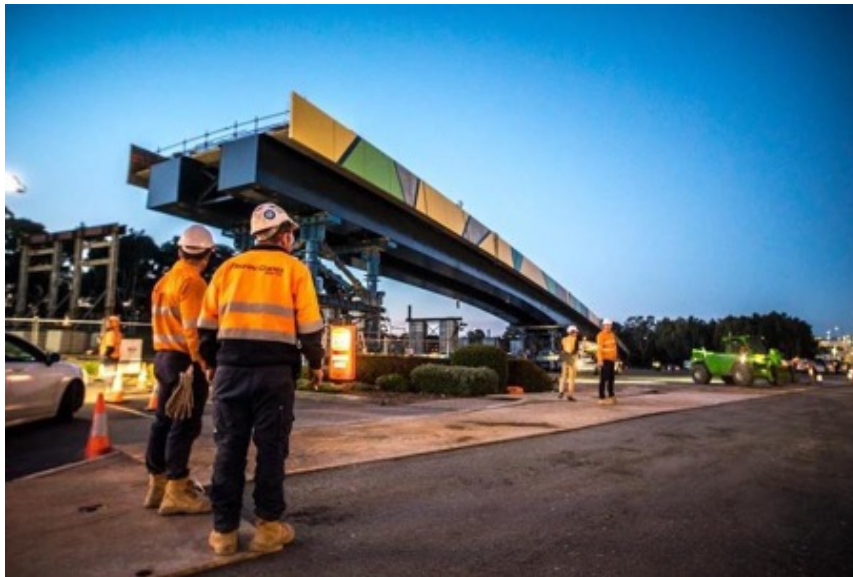
Bowhill constructed steel bridge girders for the Darlington Upgrade.
