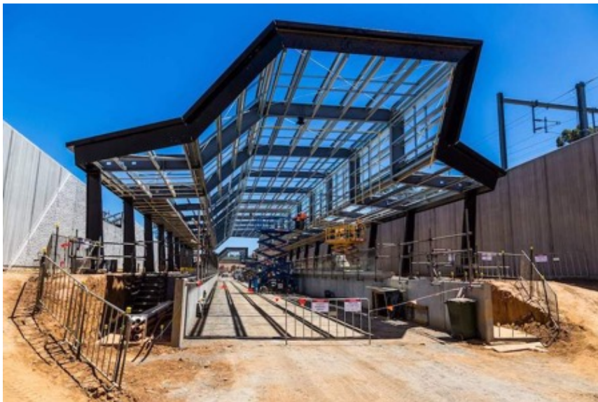
The Oaklands Crossing is also one of Bowhill Engineering's big projects.
